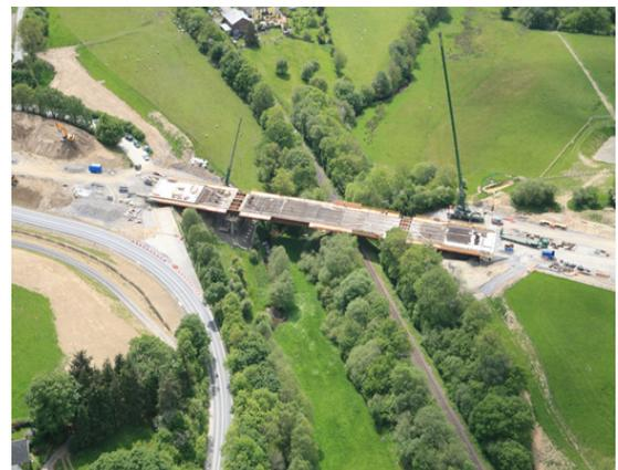
The Cwmbach Bridge crosses the Central Wales line just North of Builth Road Junction, near Builth Wells. The structure comprised a three span bridge, with reinforced concrete abutments at each end and two centrally located reinforced concrete piers, the over deck was a structural steelwork concrete composite.
